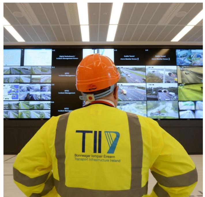
The 52 x 55" MultiSync® UN551S ultra-narrow bezel displays configure to create a video wall 13 screens wide by 4 high, with only the smallest image gap at just 1.8mm. *"The NEC display has an extremely narrow frame which gives us maximum screen area for the video wall with minimal interruption to the image,"* explains Darren Byrne, project director at ERTO. *"Image quality and reliability is essential for our operations and we are very confident in the NEC displays."*
